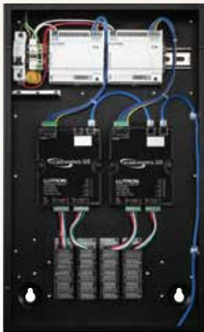
21" Low Voltage Enclosure
