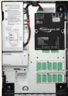
14" Low Voltage Enclosure
